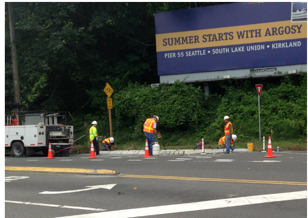
Installing a wheel curb to protect bicyclists in the bicycle lane from sharply turning traffic.
