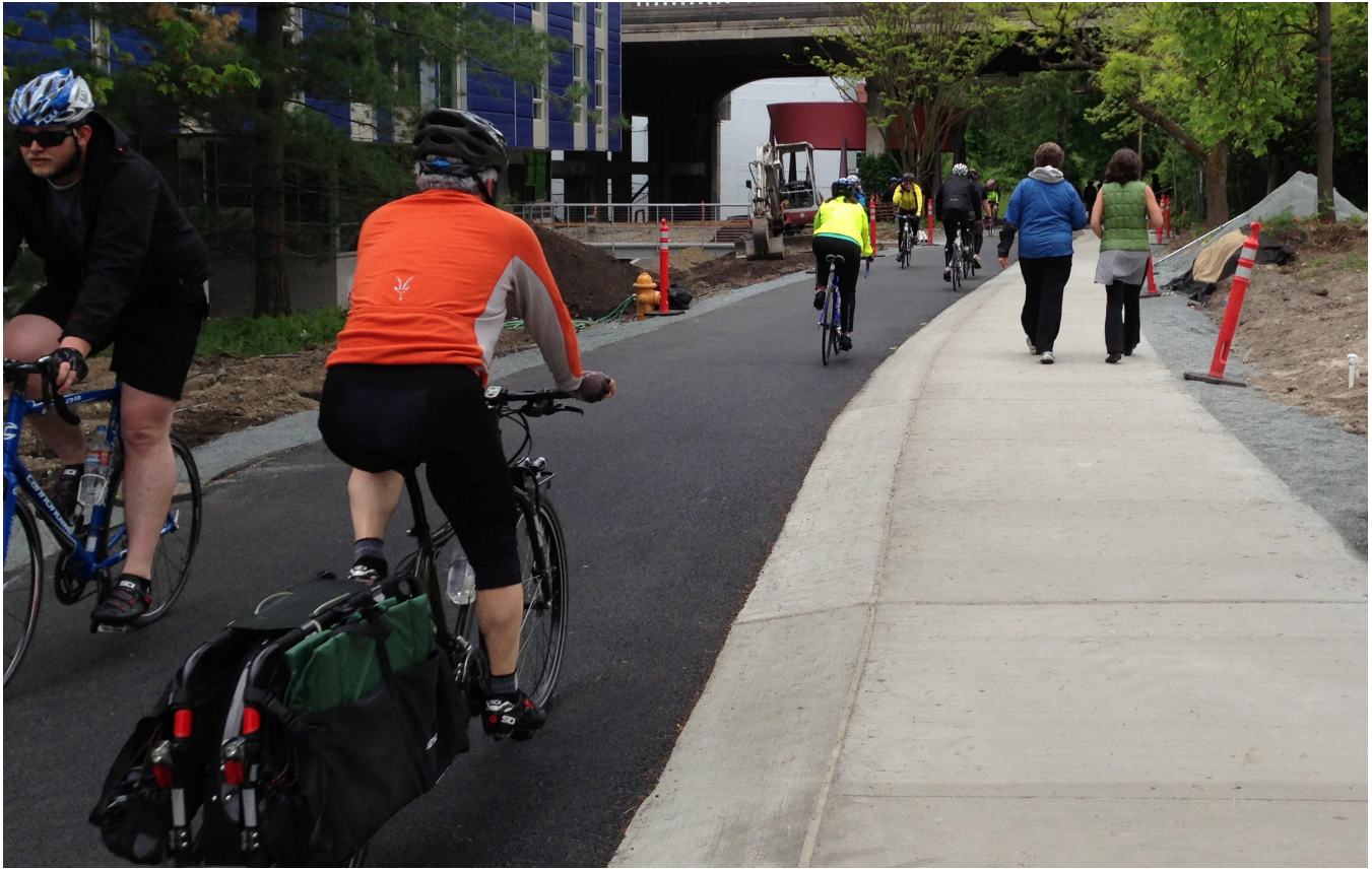
A recently renovated segment of the Burke-Gilman Trail on the University of Washington Campus provides separate space for bicyclists and pedestrians.
